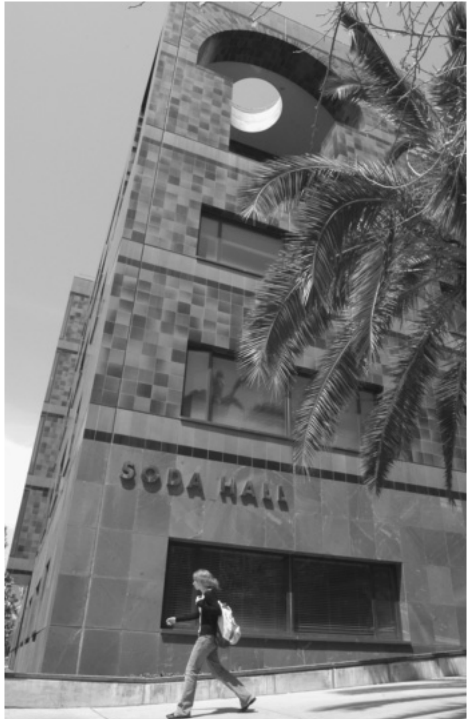
▲ In Soda Hall (above), “the building is the computer,” with advanced networking, wireless, and access to computer clusters for shared computing power. The building was designed to foster a team approach to computing innovation and houses classrooms and labs dedicated to computer science.
