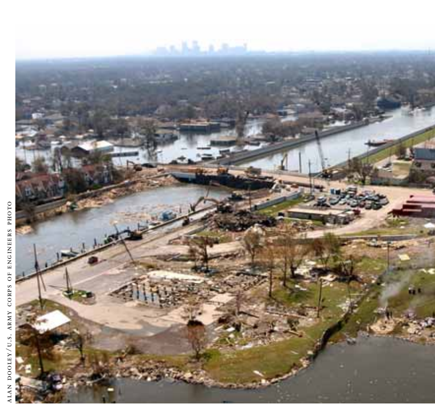
The levees keeping Lake Pontchartrain out of New Orleans, an example of the inadequate infrastructure described in ASCE's report, were particularly vulnerable to Hurricane Katrina. Here, a breach in the 17th Street Canal is visible in the upper right-hand corner. The New Orleans skyline lies in the distance.
